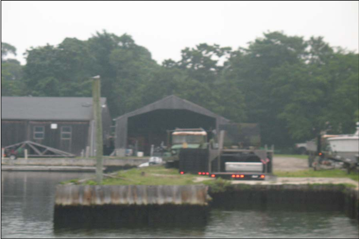
Photo 5: View of industrial parcel on Patchogue River.
